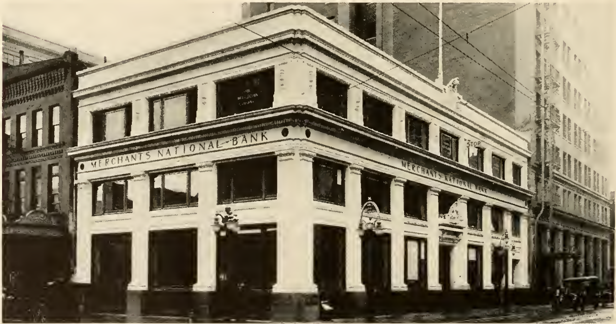
MERCHANTS NATIONAL BANK, PORTLAND, ORE.
